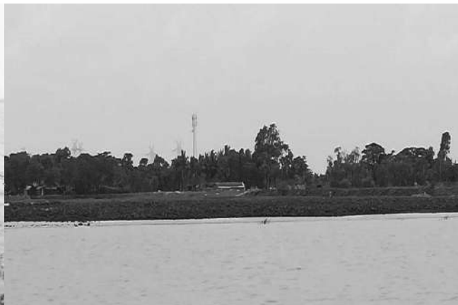
Bank Protection (Phase-I) at Shalukkhali
