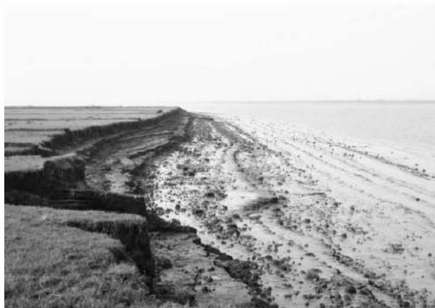
Erosion at Shalukkhali
